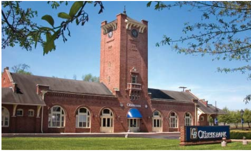
Train Station Office in Downtown Kingsport
